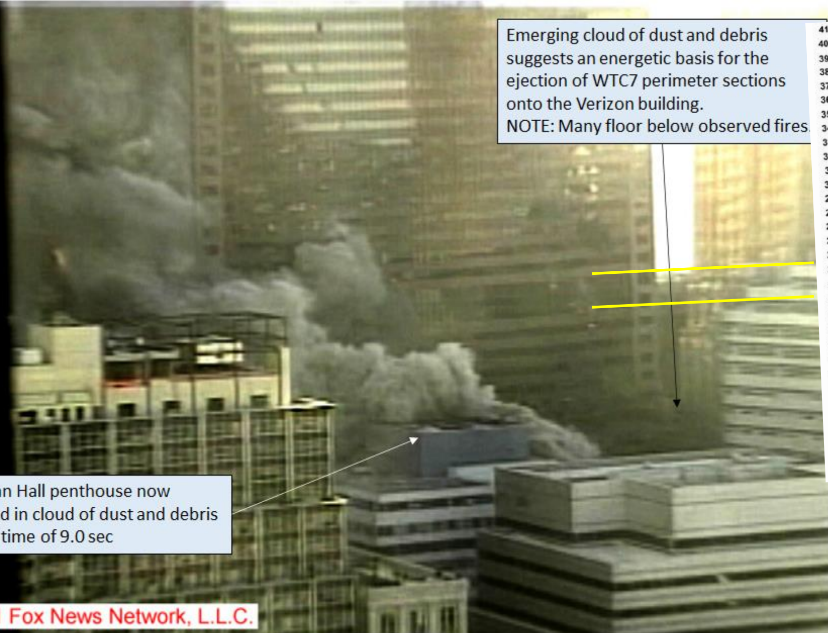
Figure 5–207. Frame from the Camera 6 video clip in Figure 5–189, showing the north face of WTC 7 9.0 s ± 0.2 s after the east penthouse began to move downward. The intensities have been adjusted.
