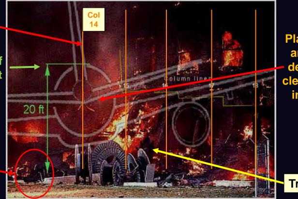
Plane impact angle of 42 degrees not clearly shown in drawing
