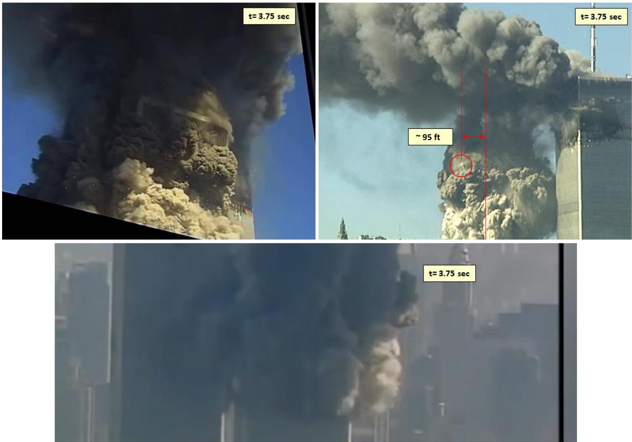
*Figure Appendix 16: At  $t=3.75$  – The east and north sides of the top of the South Tower are visible in the “Reviere” and “DeJong” videos, respectively. At this time the corner of the South Tower is approximately 95 feet over the east edge of the South Tower. At this distance from the tower, gravity-only forces could not dismember this corner and the corner should have remained visible as it plummeted to the ground. But instead, it was dismembered by other, propellant, forces.*
