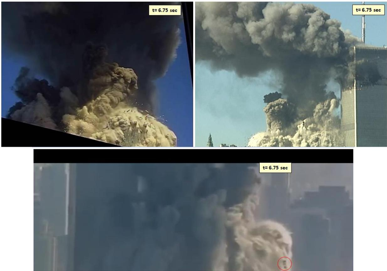
Figure Appendix 28: At t=6.75 – Perimeter columns are clearly seen in the “Reviere” video and top of the columns remains visible in the “DeJong” video. These perimeter column sections are captured in the “unnamed” video.
