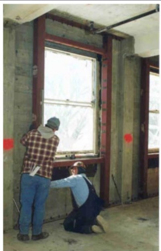
Workers in Wedge 1 install framework that will strengthen the walls around new blast-resistant windows.
