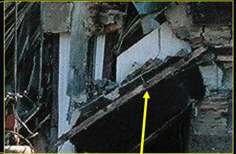
Through-bolt connection
